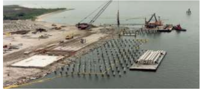
Figure 57. Construction on pylons
