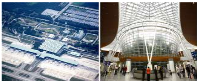
Figure 168. Kuala Lumpur International Airport (KLIA), (Bahasa Malaysia: Lapangan Terbang Antarabangsa Kuala Lumpur). (Architect: Kisho Kurokawa, 1998)
