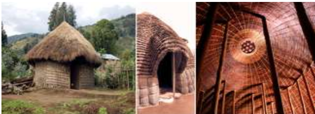
Figure 157. Traditional dwellings in Rwanda, Africa Source: http://www.africavernaculararchitecture.com/rwanda/ , Accessed: July 6, 2023. Source: http://www.africavernaculararchitecture.com/wpcontent/uploads/2015/04/Rwanda-Kings-Hut-interiorsubmitted-by-Larsen-Pay%C3%A113.jpg , Accessed: July 6, 2023.
