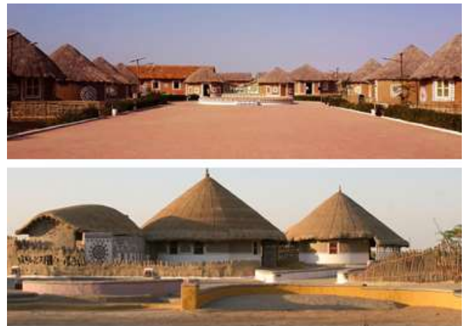
Figure 141. Bhunga houses in the desert areas of Kutch, Gujarat state, western India
