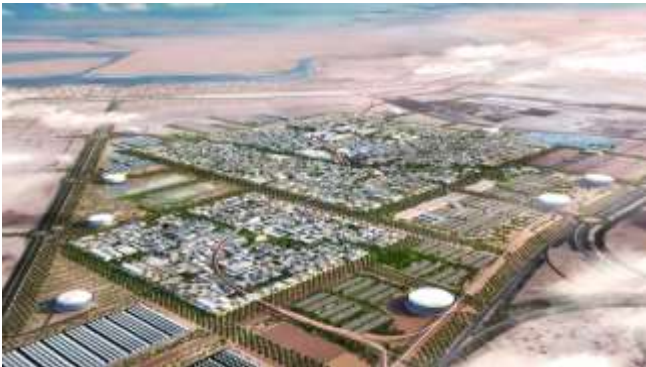
Figure 174. Masdar City (Arabic: مصدر مدينة), Abu Dhabi (Architects: Foster + Partners, 2006)
