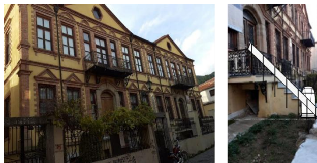
Figure 2. Proposed ramp solution for the main entrance of Kuyumcuoğlu Mansion (Xanthi Folklore Museum), Greece. Source: Authors.
