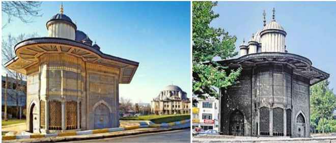
Figure 62. Azapkapı Saliha Sultan Fountain
