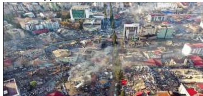
Figure 8. View Kahramanmaraş Metropolitan Presidency Service Building after the earthquake, © gazetedogu, available at https://www.gazetedogu.com/iste-kahramanmaras-in-merkezi/7455/
