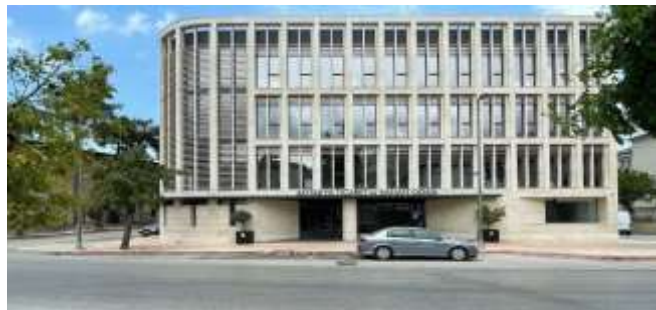
Figure 6. Antakya Chamber of Commerce and Industry and general views of the building. © Ömer Selçuk Baz, Published by Çinici Mimarlık's website in the public domain, available at https://www.cinicimimarlik.com/tr/antakya-ticaret-ve-sanayi-odasi-yonetim-binasi/
