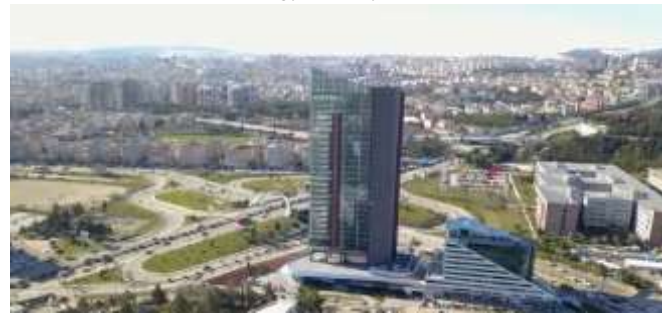
Figure 7. General views of the Koluman Tower, published on Koluman Tower's website, in the public domain, available at https://koluman-tower.com/
