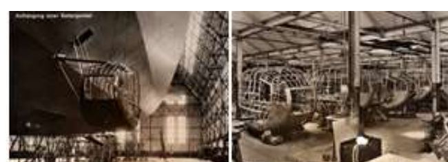
Figure 67. Left: One of the Graf Zeppelin's two port engine nacelles, under construction. Right: Five nacelles of the Graf Zeppelin under construction
