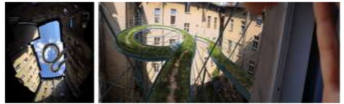
Figure 140. A walking balcony suspended in the middle of a dark courtyard, Gliwice, Poland, 2015 (architects: Zalewski Architecture Group)
