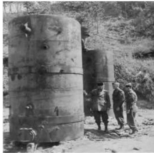
Figure 122. Rusted hydrogen production tanks are all that remain of a former balloon launch (US Army photo, SC 284185)
