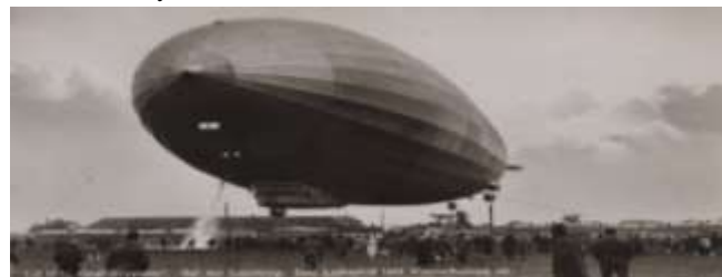
Figure 66. LZ-127 Graf Zeppelin drops water ballast during landing
