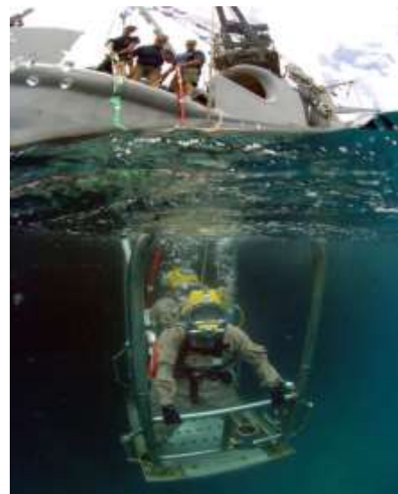
Figure 30. Divers ride on a stage to an underwater workplace Source: https://en.wikipedia.org/wiki/Underwater_diving , Accessed: July 9, 2023
