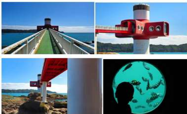
Figure 62. Ashizuri Underwater Observation Tower, Tatsukushi Marine Park, Kochi Prefecture, Japan, 1971 (Architect: Yoshikatsu Tsuboi)
